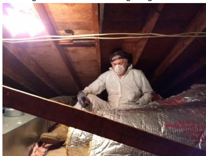
Dan adding the ductwork insulation
